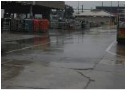
Vehicle Loading Bay – No controls.
